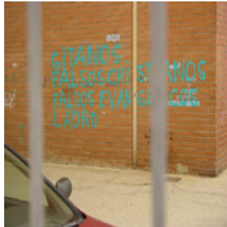
Photo 4.3 – vandalism in the Old Mina
