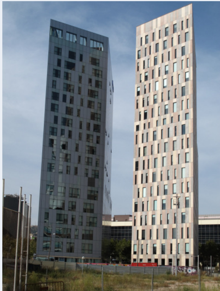
Media Park development in the 22@ district of Poblenou
