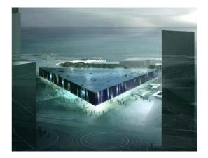
The main structure of the platform is the roof, a 3.5m height macro-structure based on a grid built of steel girders and covered by two pos-tensed concrete flagstones. The platform's façades are actually structural beams, supporting the lower flagstone in order to keep it free of columns, generating a diaphanous space in the interior of the platform as well as at ground level.
